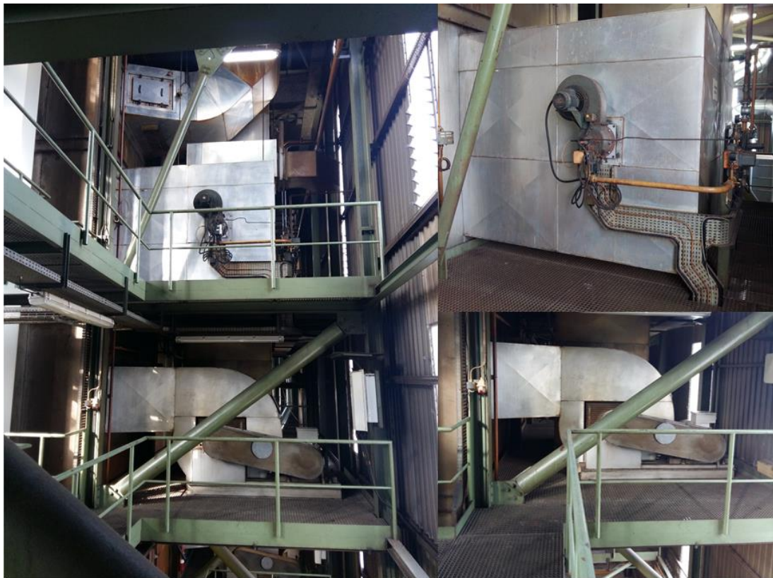
Figure 33. Burner with bottom and top ventilations.
