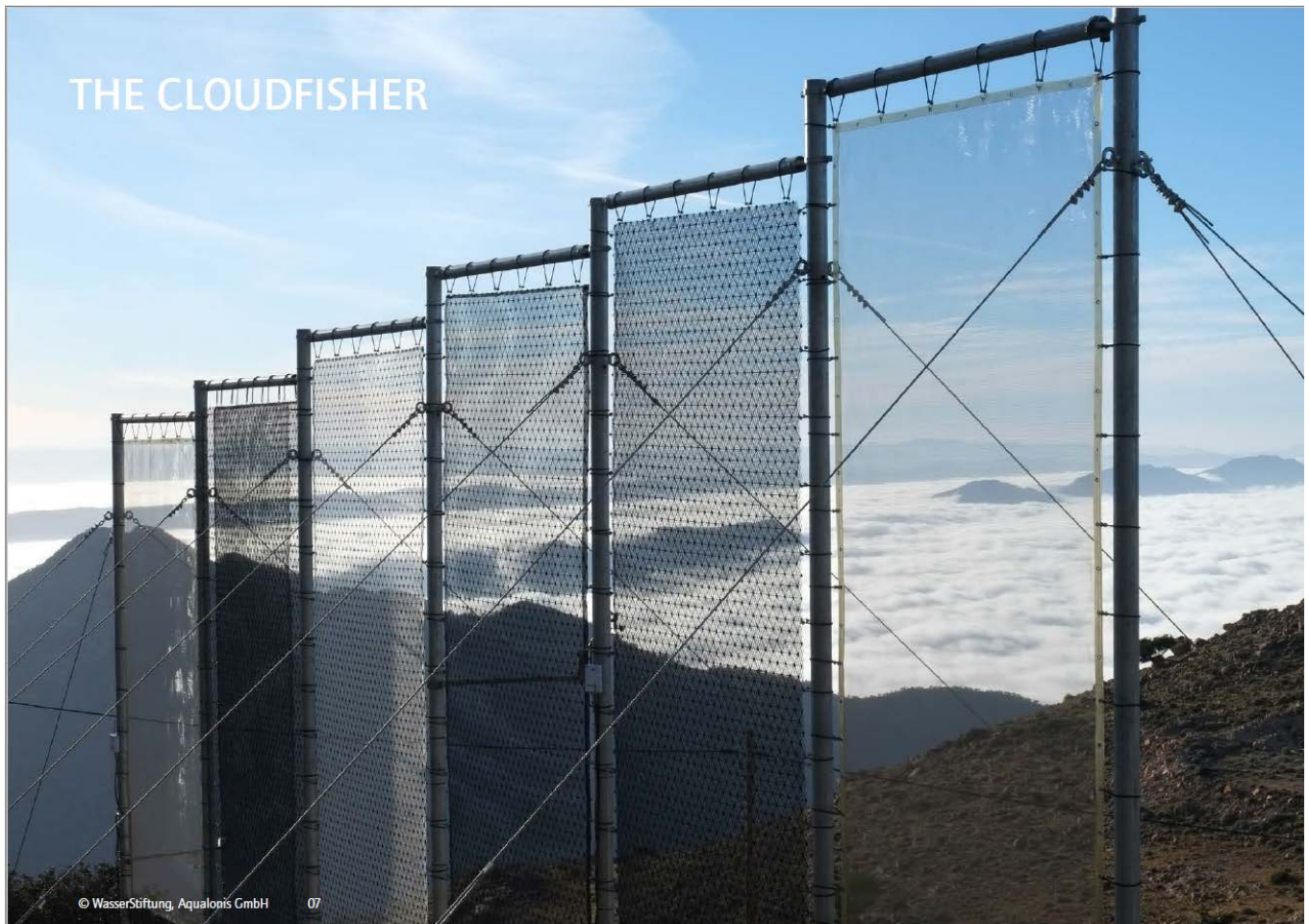
Figure 1: Fog nets installed by Dar Si Hmad (Trautwein, 2015)
