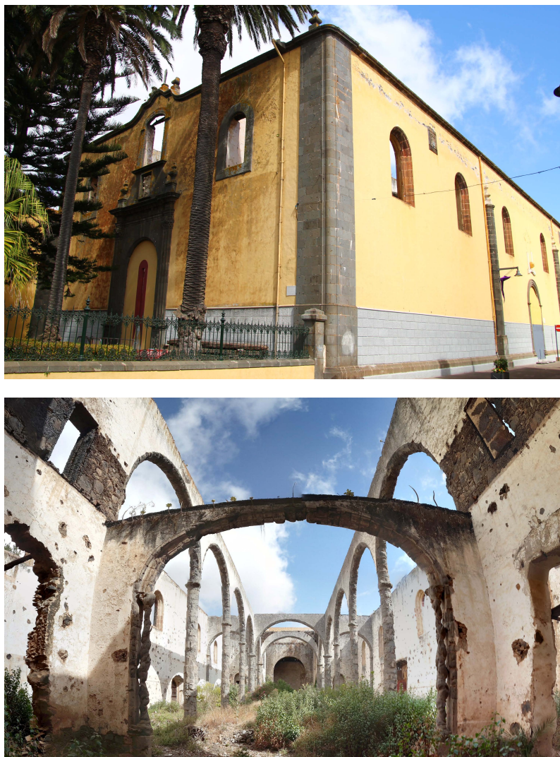
FIGURE 3. Main facade and walls of the church of San Agustín, next to the old convent of the same order, in its present state after a fire in 1964 consumed its interior and collapsed the roof. Its location marked the southeastern boundary of the old town, until the Lower Town was built (photographs by the authors).
