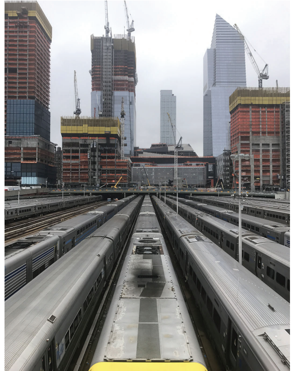
Fig.2: Commuter rail trains below the platform and view of the construction site for Hudson Yards. Source: photo by Nicola Pisacane.
