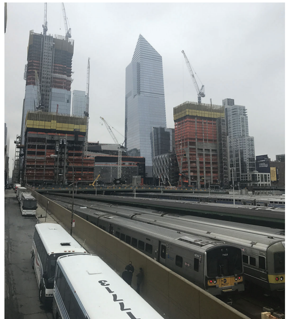
Fig.3: View of the construction site from the High Line. Source: photo by Nicola Pisacane.
