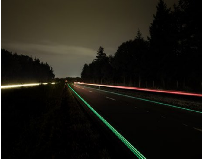
Fig. 6. Road marking glowing in the dark [43].
