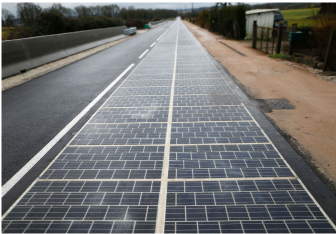
Fig. 3. Photovoltaic road in France [38].
