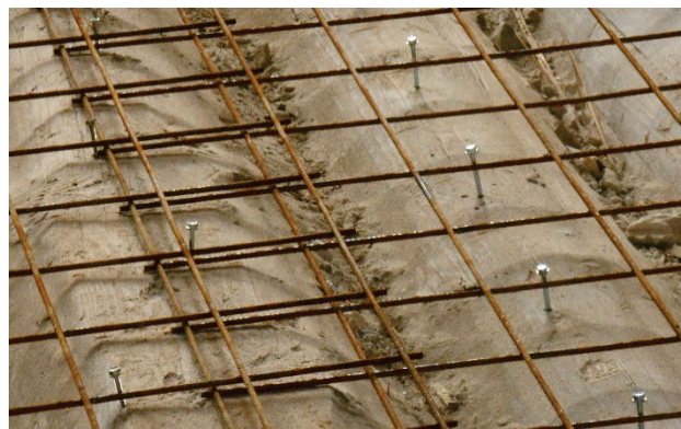
Figure 14 Connecting system head screw d=10 mm
