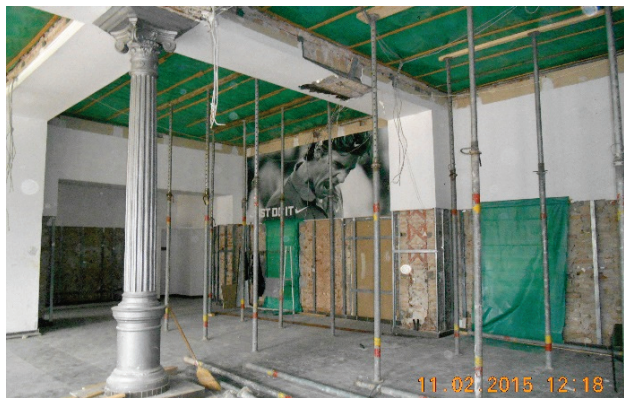
Figure 12 Scaffolding structure under timber floor
