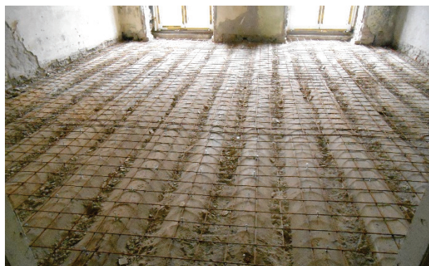
Figure 13 Rounded timber beams and reinforcement mesh
