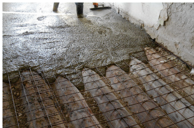
Figure 15 Erection of composite timber–concrete floor
