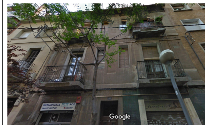
Photograph of the building
