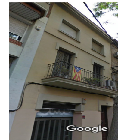
Photograph of the building
