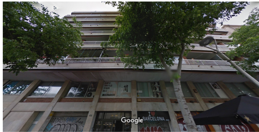
Photograph of the building
