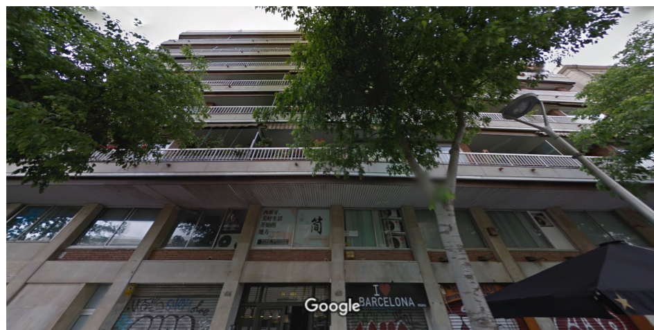
Photograph of the building
