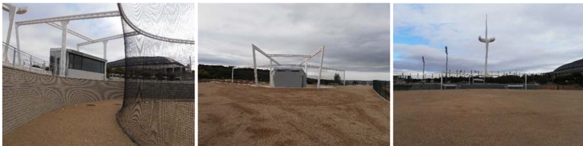
Figure 10. Photographs finally works on phase 1
