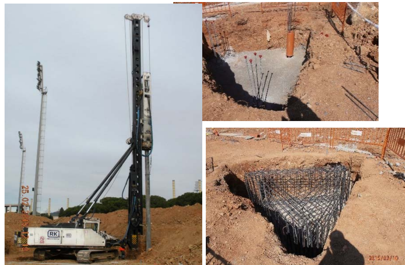
Figure 6. Photographs of the execution of the foundation
