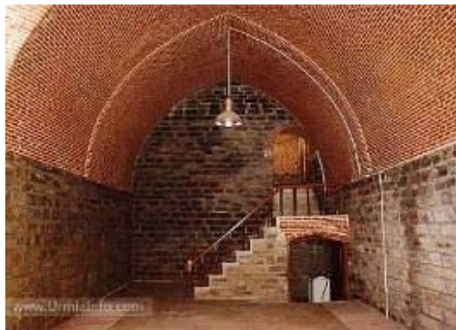
Fig.12. Nine stairs ice-house in Oroumiye, Azarbayjan( after repair)
