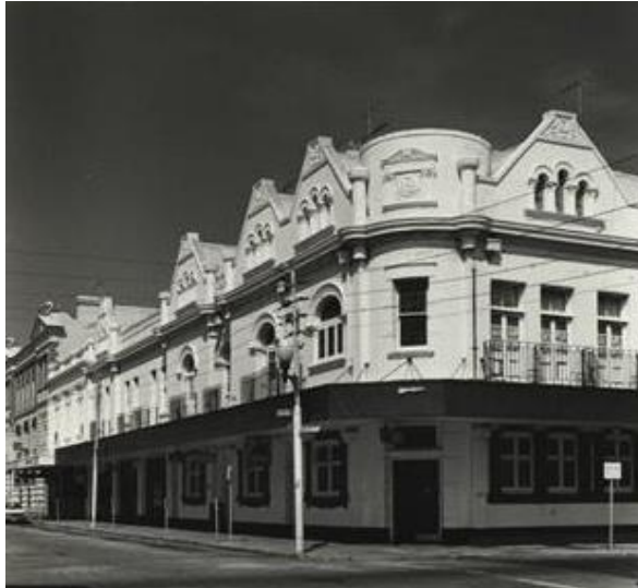
Figure 4.15 F.A. Sharr, Front corner elevation . 1981, Image. Reproduced from: Heritage Council: State Heritage Office.
