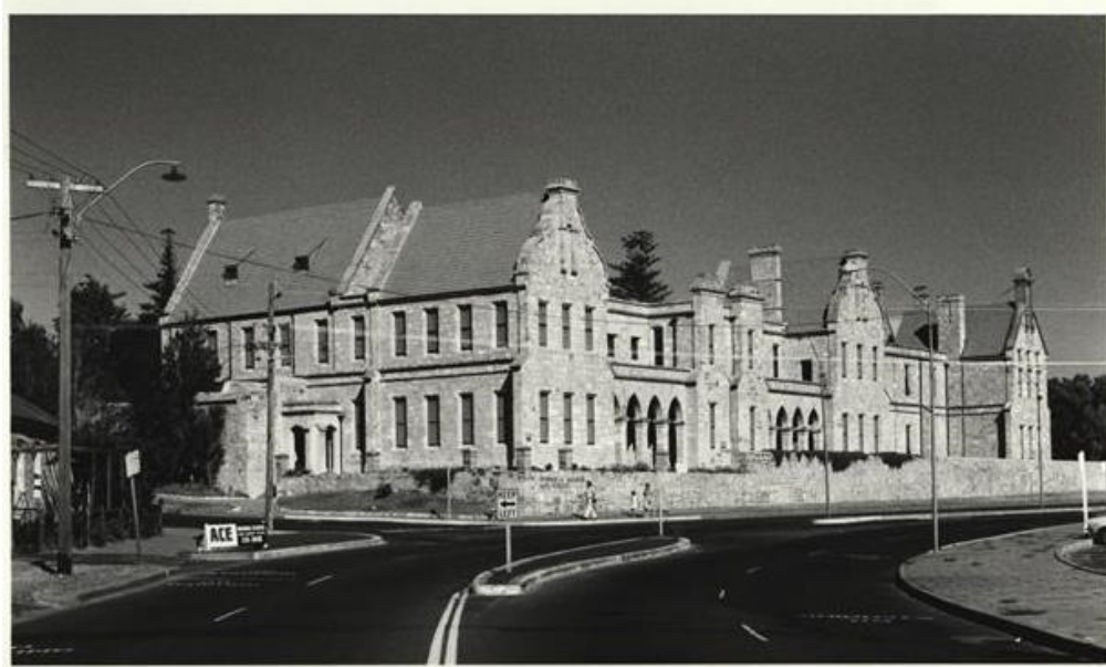
Figure 4.7 F.A. Sharr, Lunatic Asylum - Corner elevation from James Street. 1981. Image. Reproduced from: Heritage Council: State Heritage Office.
