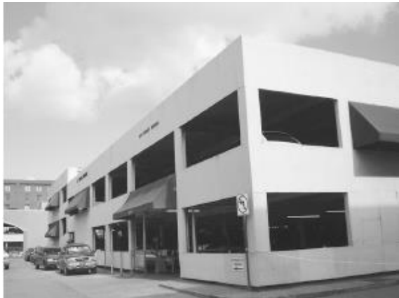
Figure 6. Parking garage in the Ellis square
