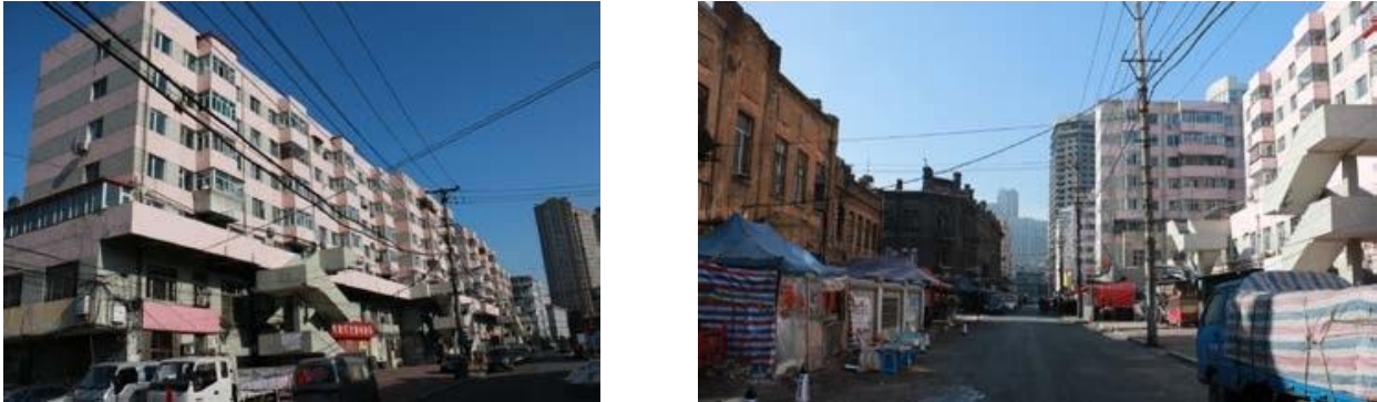
Figure 20. New residential buildings
