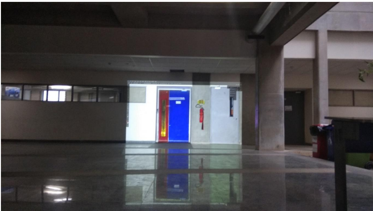
Figure 50 Surface 5 Academic block ISAC gate
