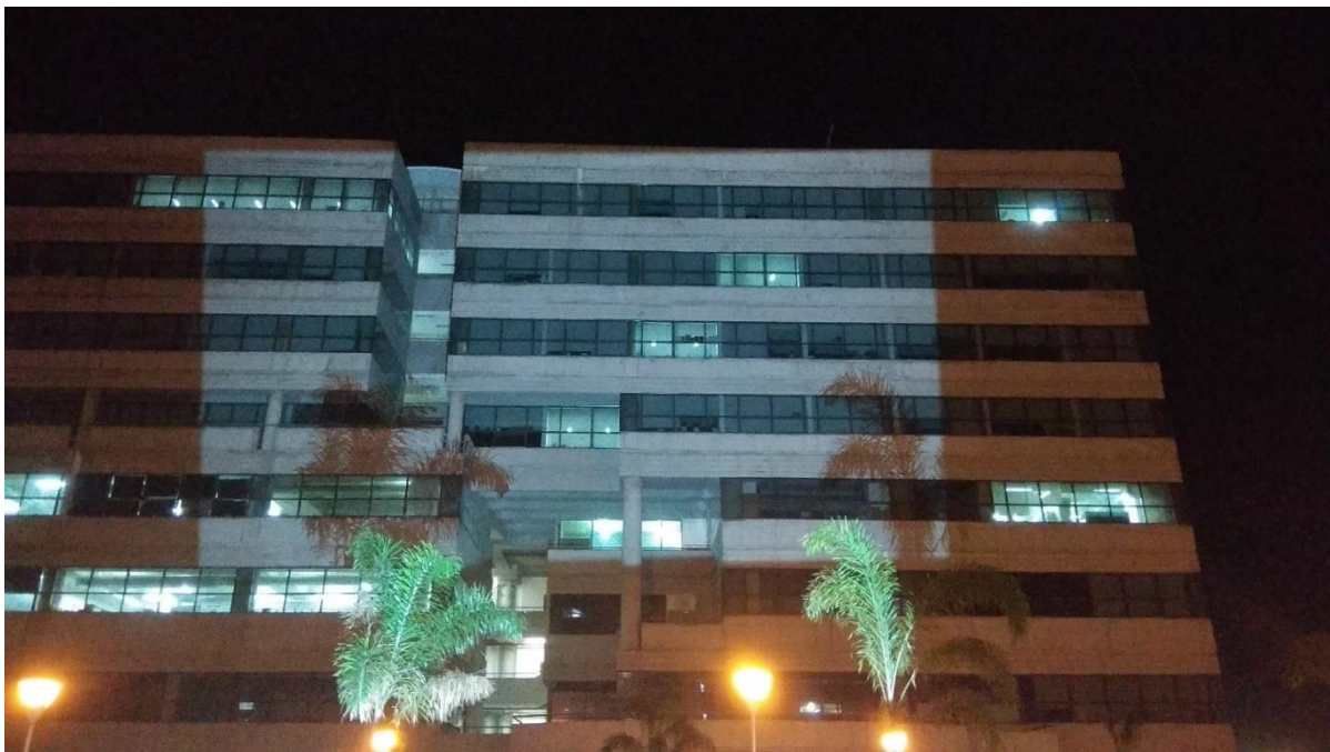
Figure 58 Surface 12 C block building
