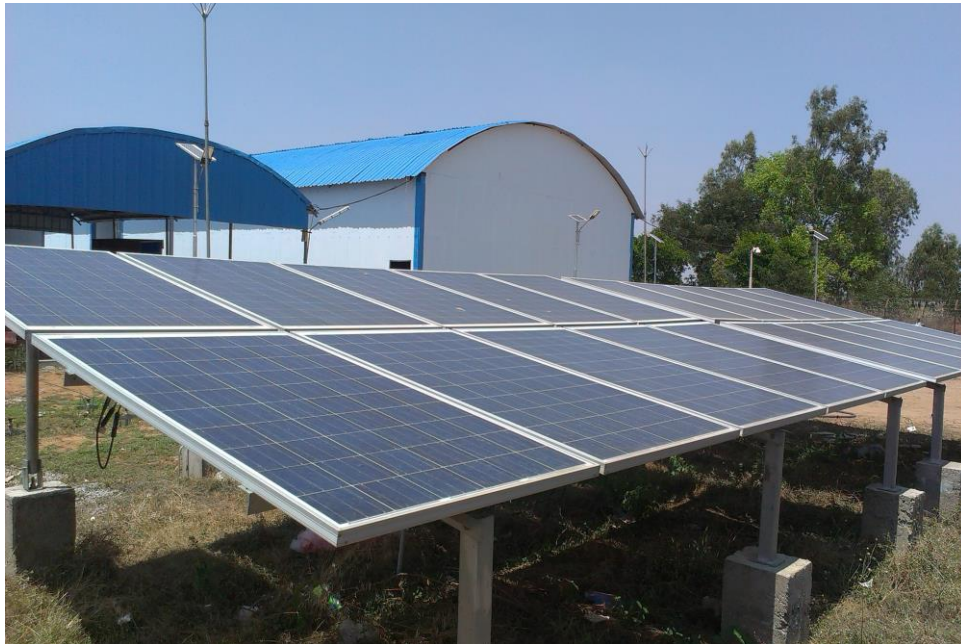
Fig.5.3 5KW off-grid PV generation system
