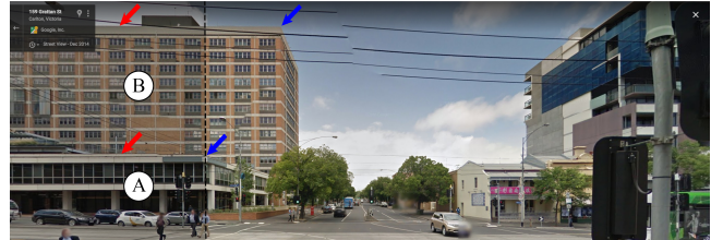
Figure 1: Building A's rooflines are hard to detect due to the overlapping with building B, while building A's corners can help figure out the true rooflines. Red arrows: building rooflines; Blue arrows: building corners.
