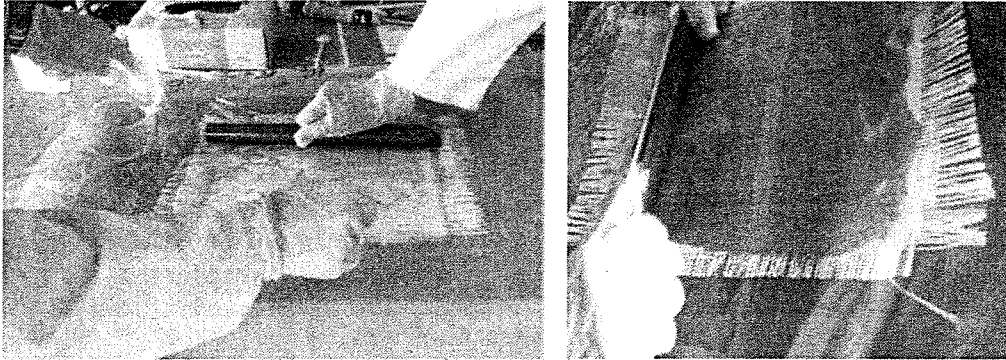
Figure 1: Application of resin on E - glass fabric
