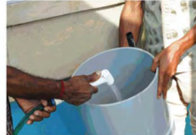
Fig.8 Cleaning the well by seawater using a spray nozzle
