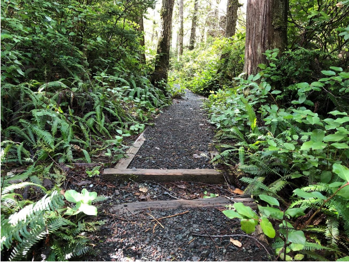
Figure 5.5. Drainage control trail infrastructure. Installed in frequent intervals along the Sand Point trail. Source: Photo by author.
