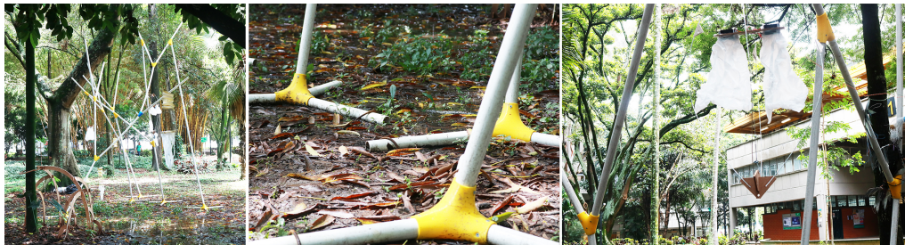
Figure 14 "Árbol de la lluvia" in front of Faculty of Architecture in Medellín University. Bars (RDE 21 PVC 1.1/4"); knots (PLA 1.75mm with printing time 5-10 hours each one)
