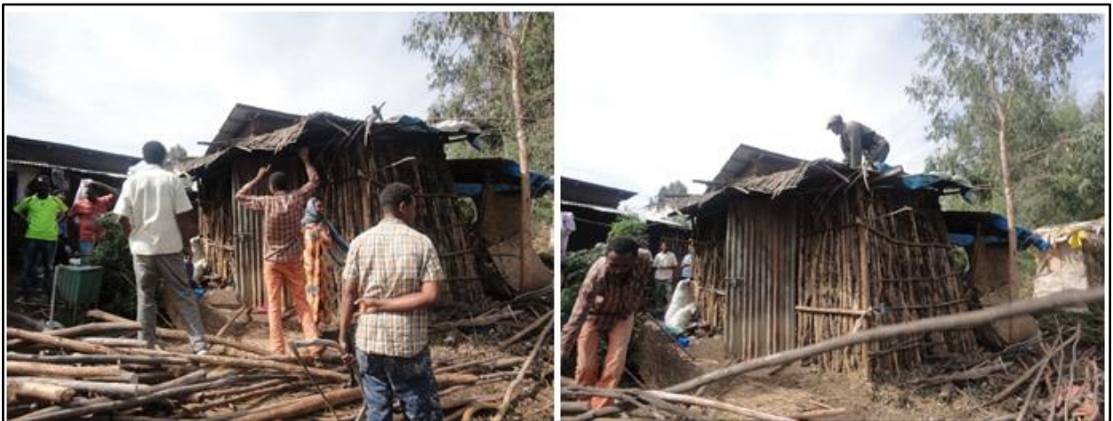
Figure 6.6: Unauthorized buildings before demolition (left) and during demolition (right)
