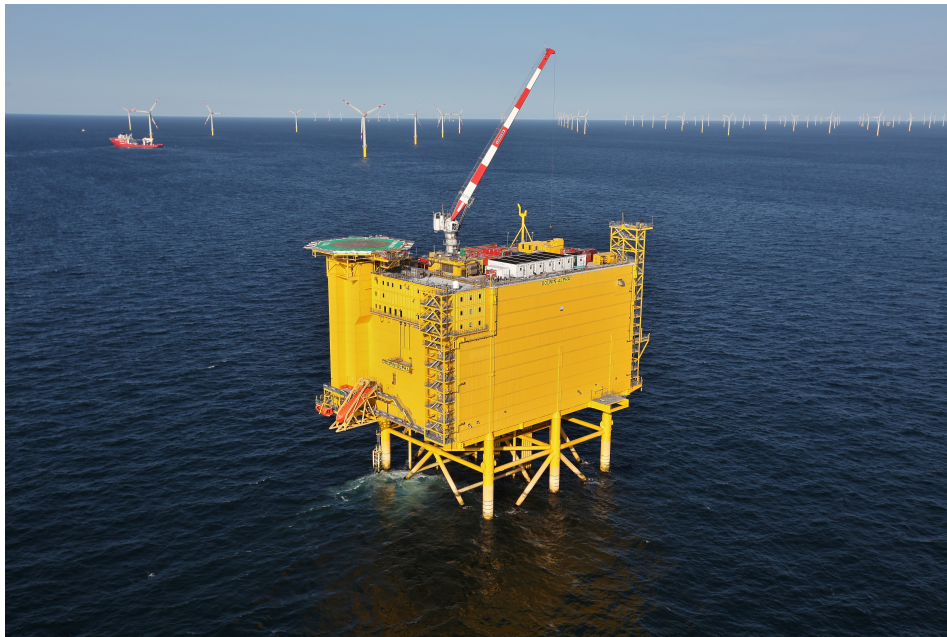
Fig. 1.3: DolWin1 offshore wind platform. Source: ABB [12].
