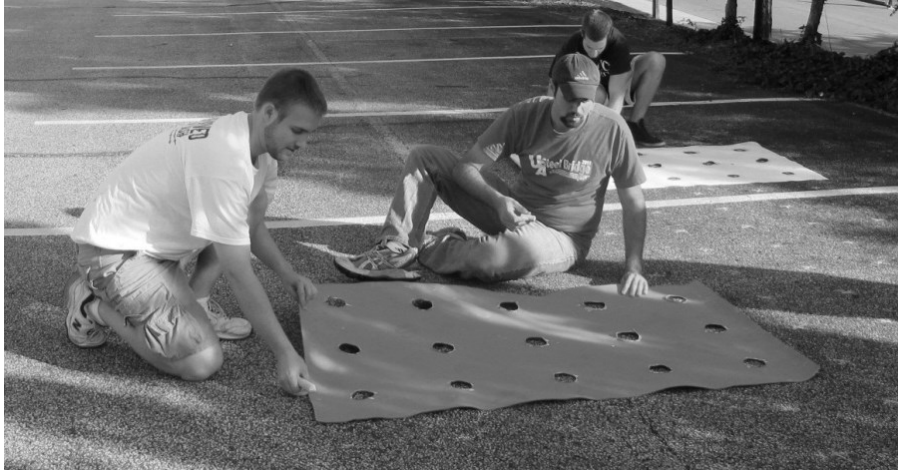
Figure 1. A template for the 1' grid of dots speeded the marking process by eliminating the need for measuring.
