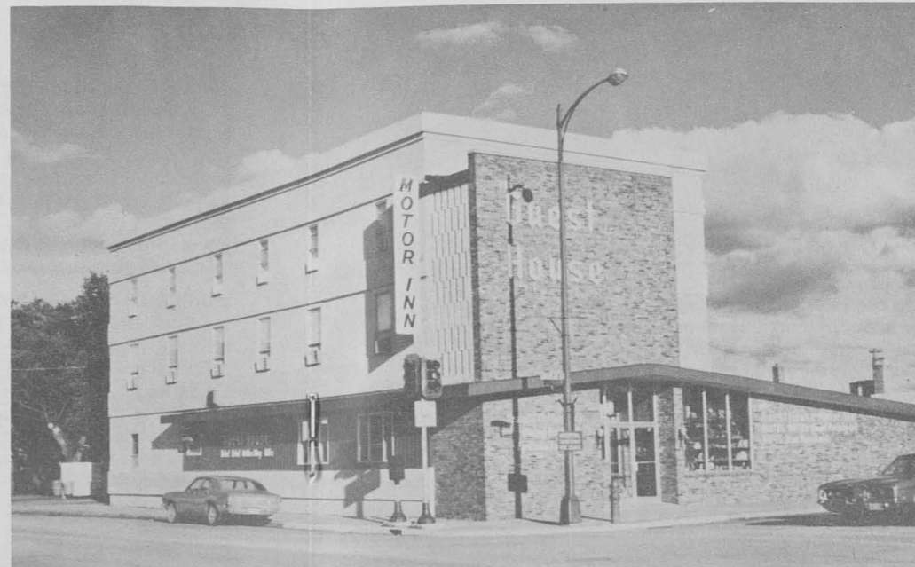
Most income from tourism comes from sales by private commercial facilities. High quality hospitality services are a must (Roseau, MN).
