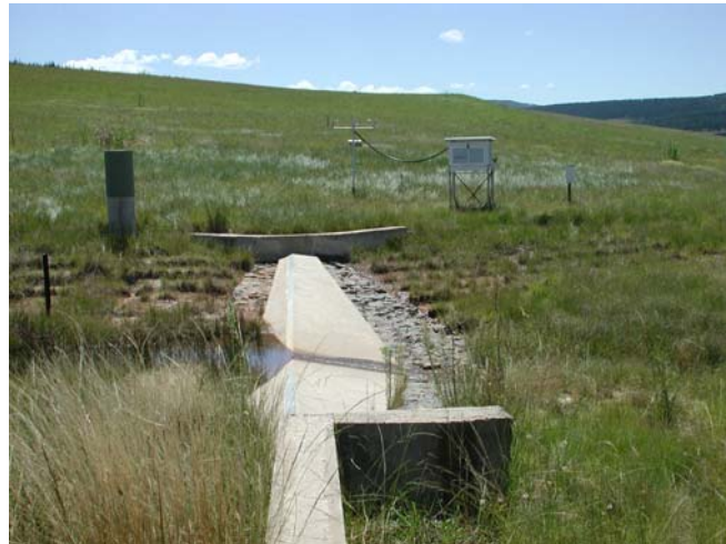
Figure 6.2: The upper weir and the full-automated weather station in the experimental test catchment Weatherley (Photograph: HELMSCHROT, 2001).
