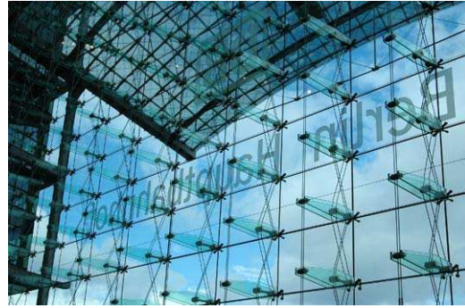
Fig. 2: Structural application of tempered glass (Glass beams, Lehrter Bahnhof, Berlin)
