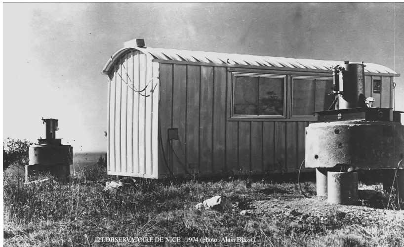
Figure 1.4: The I2T built by Labeyrie and collaborator at the Nice Observatory in 1975. It is possible to see the two small telescopes that were used to collect the first fringes of the interferometer.
