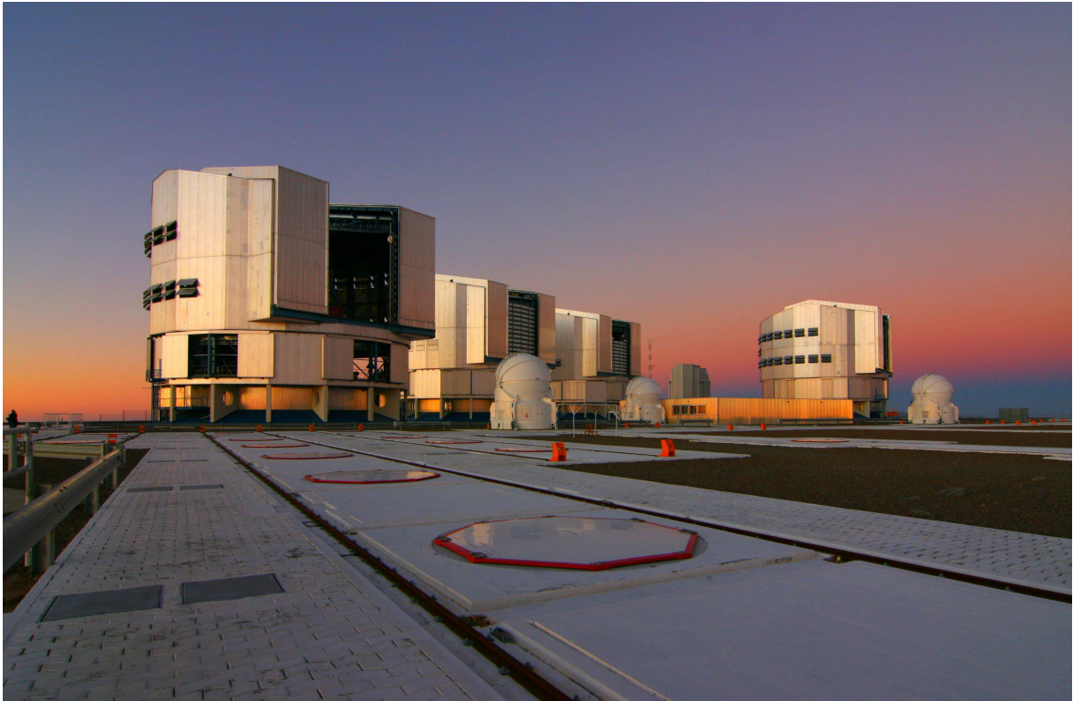
Figure 2.4: Panoramic view of the VLTI at Cerro Paranal. Four UTs and three ATs are visible. Some of the station where the ATs can be positioned are also visible.
