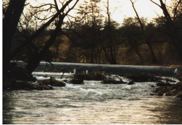
Fig. 2. The first weir is situated at the main stream of the Stream Ilm. The water flow passes the barrier atop the wall.
