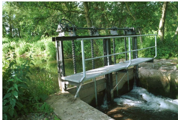
Fig. 3. The second weir is situated at a tributary of the stream. The water flow passes underneath the wooden gates
