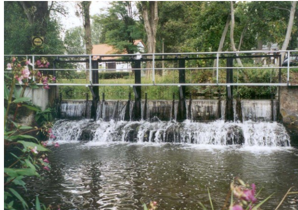
Fig. 4. The third weir is situated at the end of the tributary. The the water flows passes underneath the gates.
