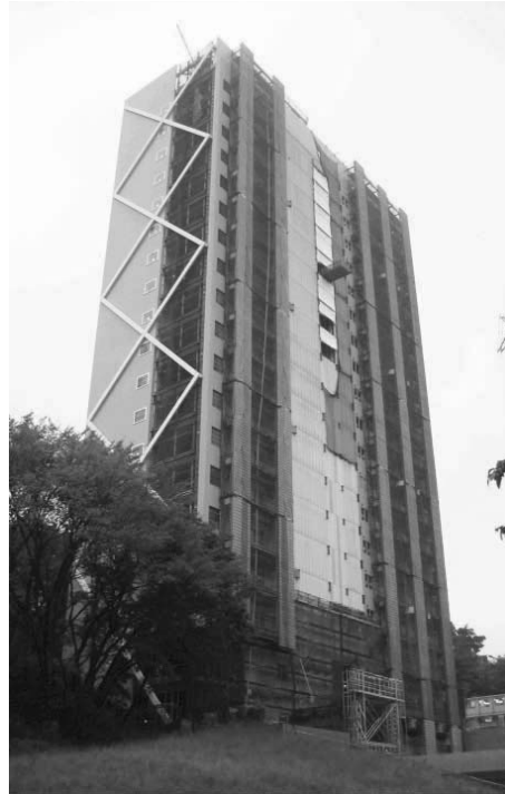
Figure 1-2 Base isolated high rise building at Tokyo Institute of Technology, Japan
