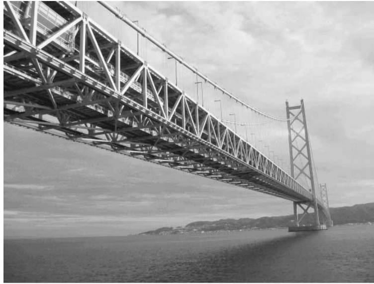
Figure 1-1 Akashi-Keikyo Bridge, Japan
