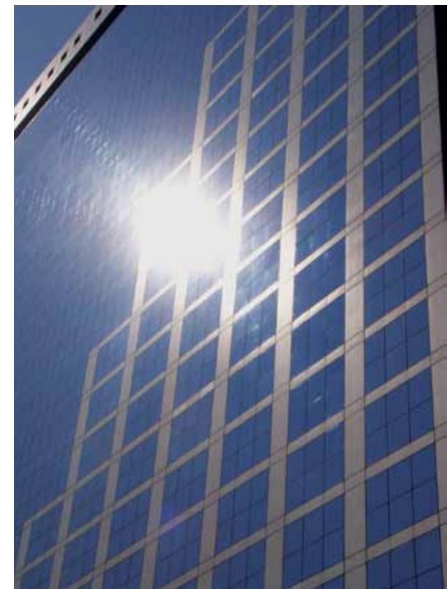
Fig. 4.7.: Highrise buildings with (mirror) glass façades causing glare, Jaragua building (above) and building at Paulista Avenue (below)
