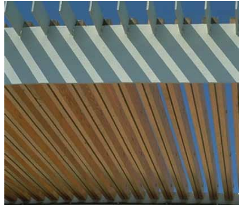
Fig. 6.1: Overhead shading elements aside from trees are pergolas, building overhangs (arcades), marquises, solar sails, canvases etc. Partially transmissive and movable device in courtyard in Seville/ Spain (Photos: Simmos Yannas)
