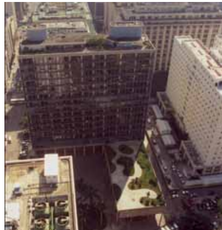
Fig. 3.14: Ministry of Education and Health (MEC) with Burle Marx's first roof gardens. Developed and constructed between 1936 and 1943 by Costa, Niemeyer, Reidy and others (left) based on ideas and sketches by Le Corbusier (right)
