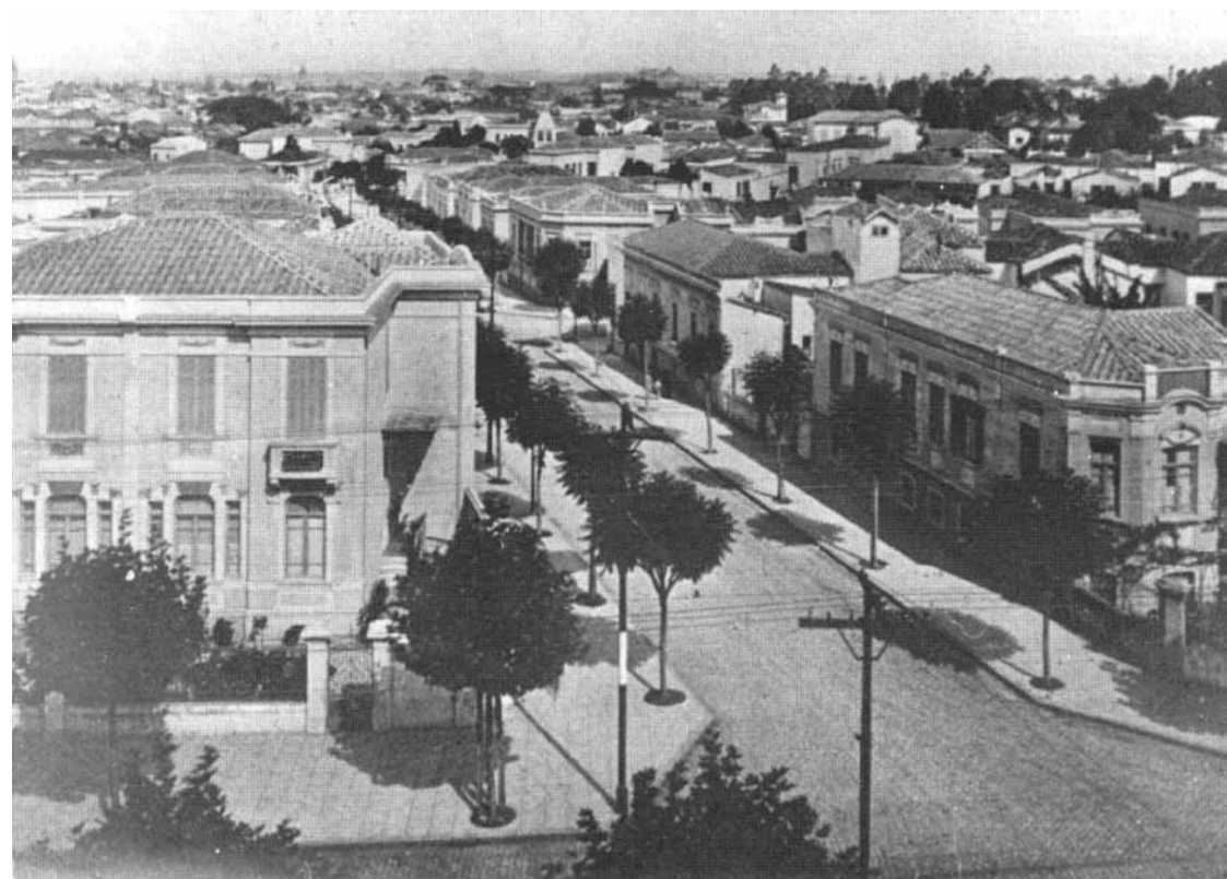
Fig. 3.6: Streets and avenues (like Avenida Angélica in wealthy districts like Higienópolis ca. 1880) received some landscaping, becoming lined with trees mostly exotic species usually planted at a distance of 5 meters, note that street trees were recently planted and cast small shadows at noon (Robba and Macedo, 2003, p. 25)
