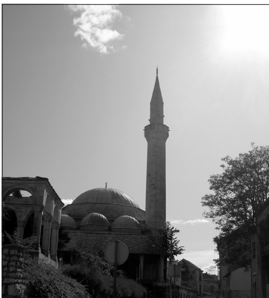
Figure 5.6: Rehabilitated Karadjozbeg Mosque.
