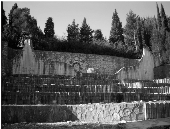
Figure 5.11: Partisan Monument Complex in complete disarray. (Source: Author)
