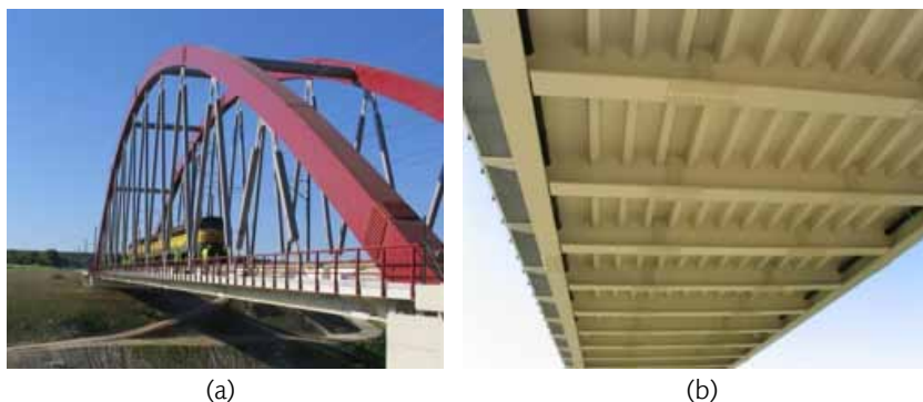
Figure 2 — Prester Bridge: a) side view and b) bottom view
