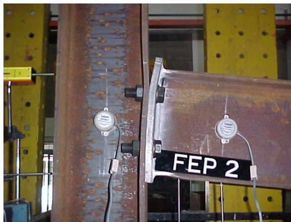
Figure 16: Failure mode of column flange and end-plate (FEP 2 connection).
