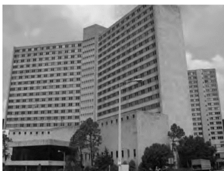
(a) Twenty-story Baptist Memorial Hospital.
