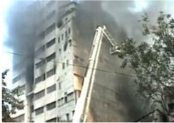
Figure 1.2-10 Fire cause partial collapse of shopping building from (Kolkata, 2013)
