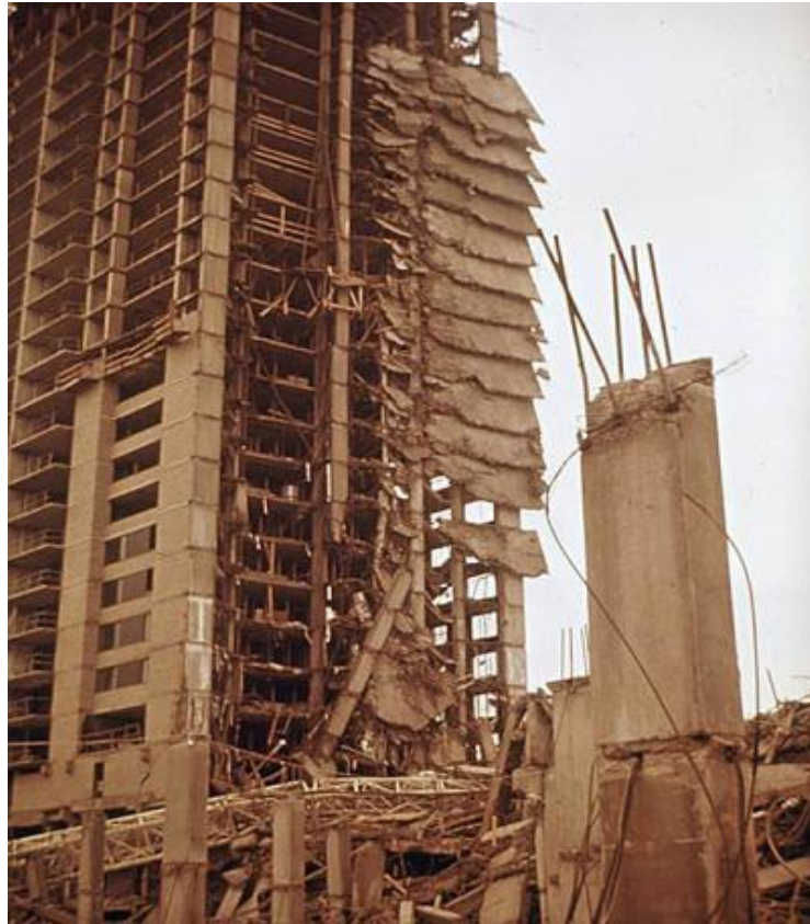
Figure 1.2-3 the federal building in the city of Oklahoma (Net World Directory, 2013)
