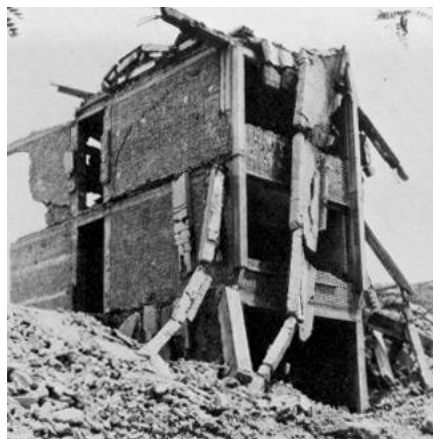
Figure 1.2-8 Partial seismic collapse of building in china from (Huixian & George W. Housner, 2016)
