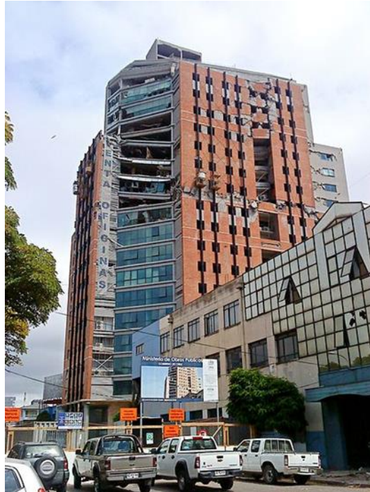
Figure 1.2-7 Partial soft-story vertical arrested collapse from (2010 Chile earthquake, 2016)
