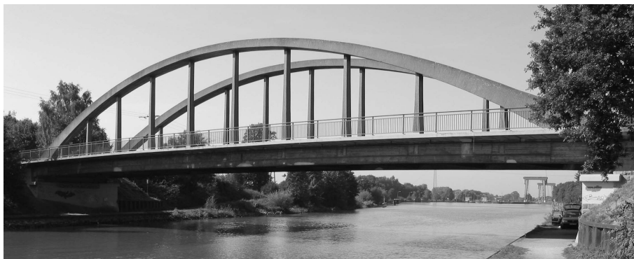
Figure 4.6: Tied Arch Bridge near by Hünxe (North Rhine-Westphalia, Germany)
