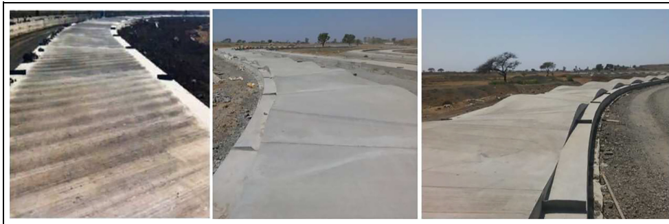
Figure 22. Some places where the tracks are not straight.
