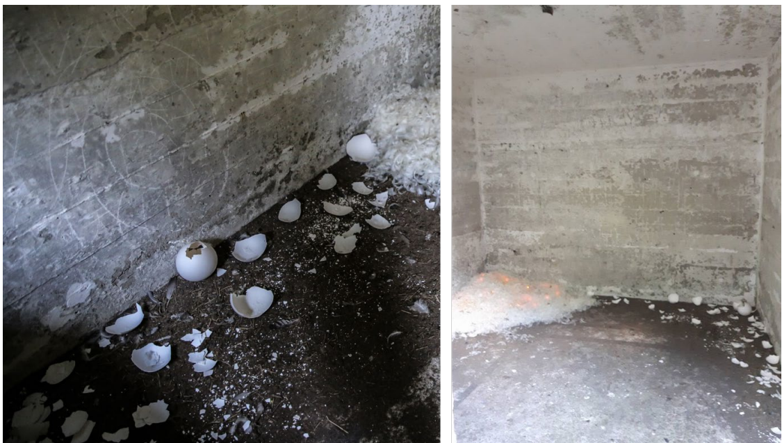
Figure 72 Broken Eggs installation
