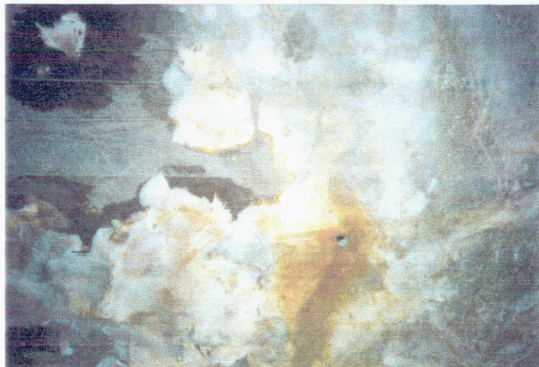
Figure 5.8 : Cord formation on floor surface. Note brown pigmentation of hyphae, brown droplets and a blue-coloured fungus growing on the dead S.lacrymans mycelia.
