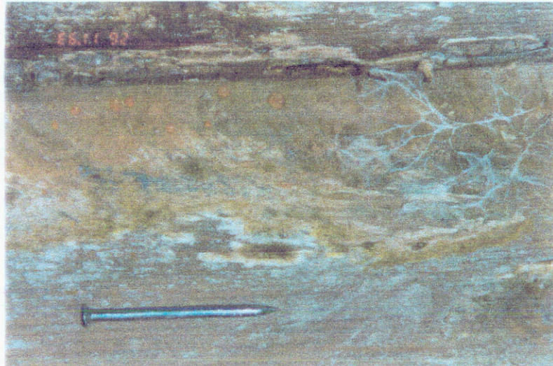
Figure 5.8 : Cord formation on floor surface. Note brown pigmentation of hyphae, brown droplets and a blue-coloured fungus growing on the dead S.lacrymans mycelia.
