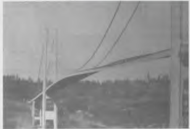
The 1940 collapse of the original Tacoma Narrows Bridge is a visually memorable example of resonance.
