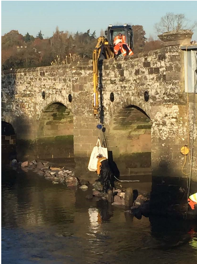
Fig 20 Rock armour installation
