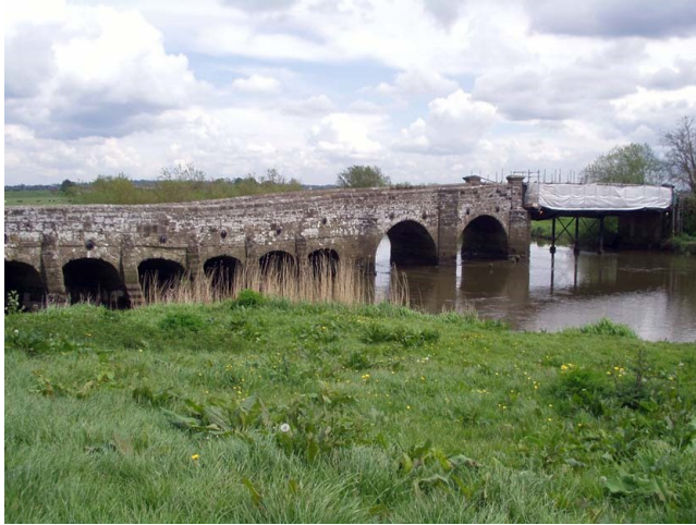
Fig 9 Extra (double) Sheeting During Repainting Operations
