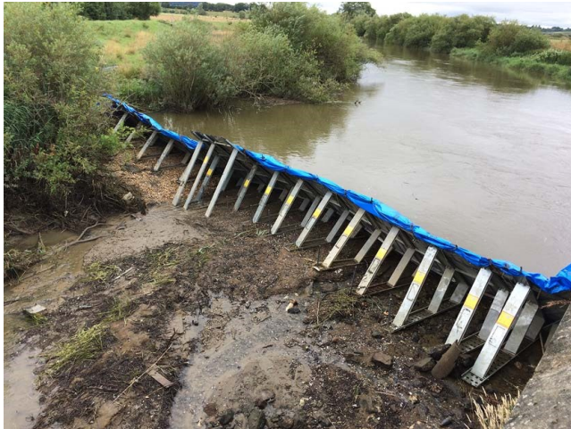
Fig 15 Temporary dam used in the early stages of the refurbishment
