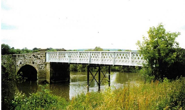
Fig 11 Greatham Bridge in 2003 after strengthening works completed
