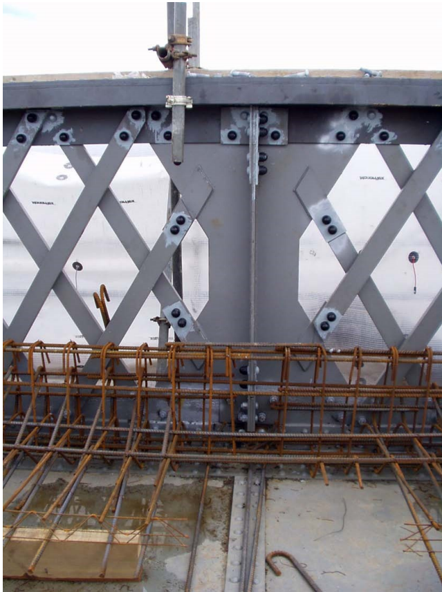
Fig 4 New design of central stiffening plate
