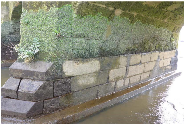
Fig 19 New masonry work
