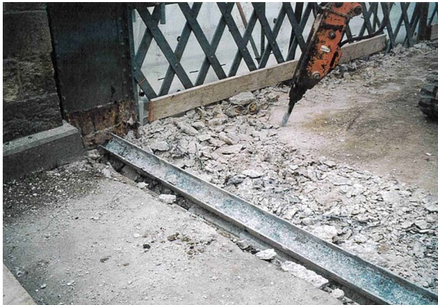
Fig 6 Original concrete deck being broken out
