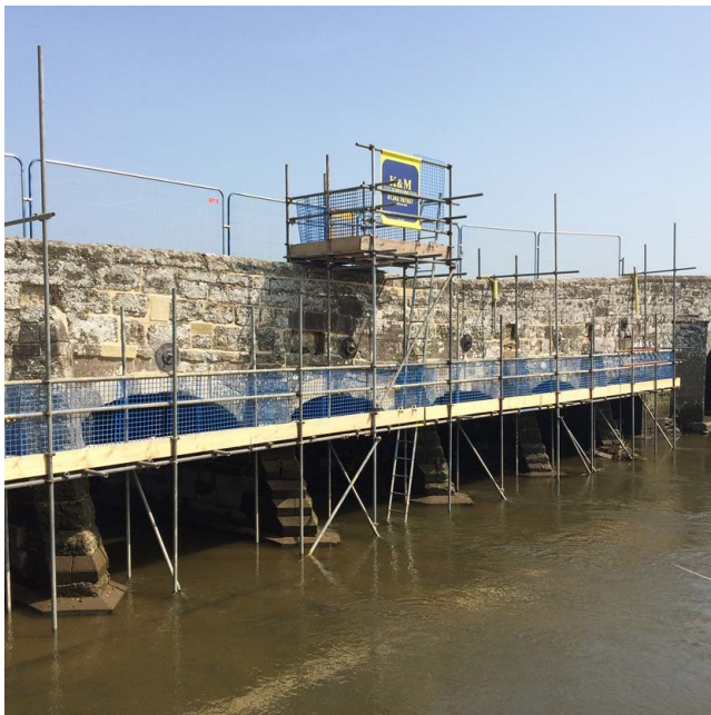
Fig 16 Refurbishment temporary works for access to arch faces
