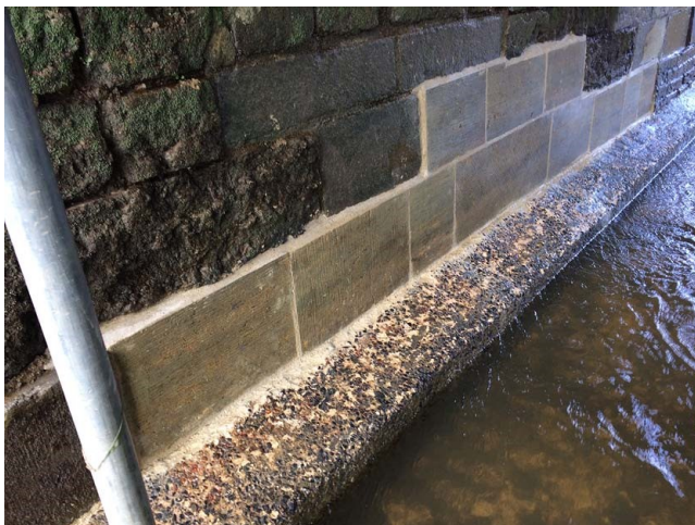
Fig 17 New masonry work
