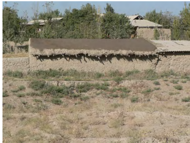
Fig 7: Barn flat roof covered with a special clay, Avazali 2012. Photo : D. Gandreau
