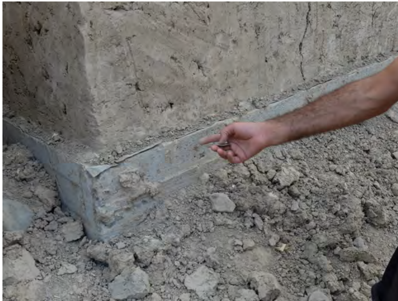
Fig 5: Concrete socle and bitumen fabric, Avazali 2015. Photo : C. Sadozai
