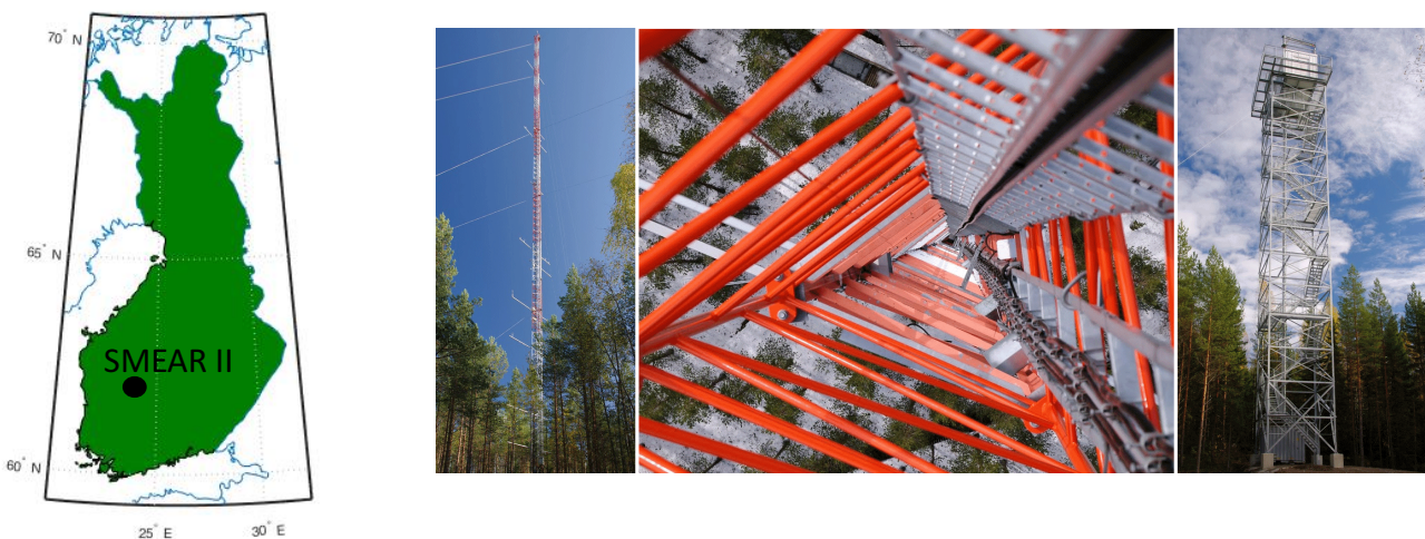
Figure 5a) Location of SMEAR II station on the map b) The measurement mast is 127 m tall, c) the view from the top of the measurement mast during winter time and d) the new radiation tower is 35 m tall (INAR (Institute for Atmospheric and Earth System Research), 2018) .
