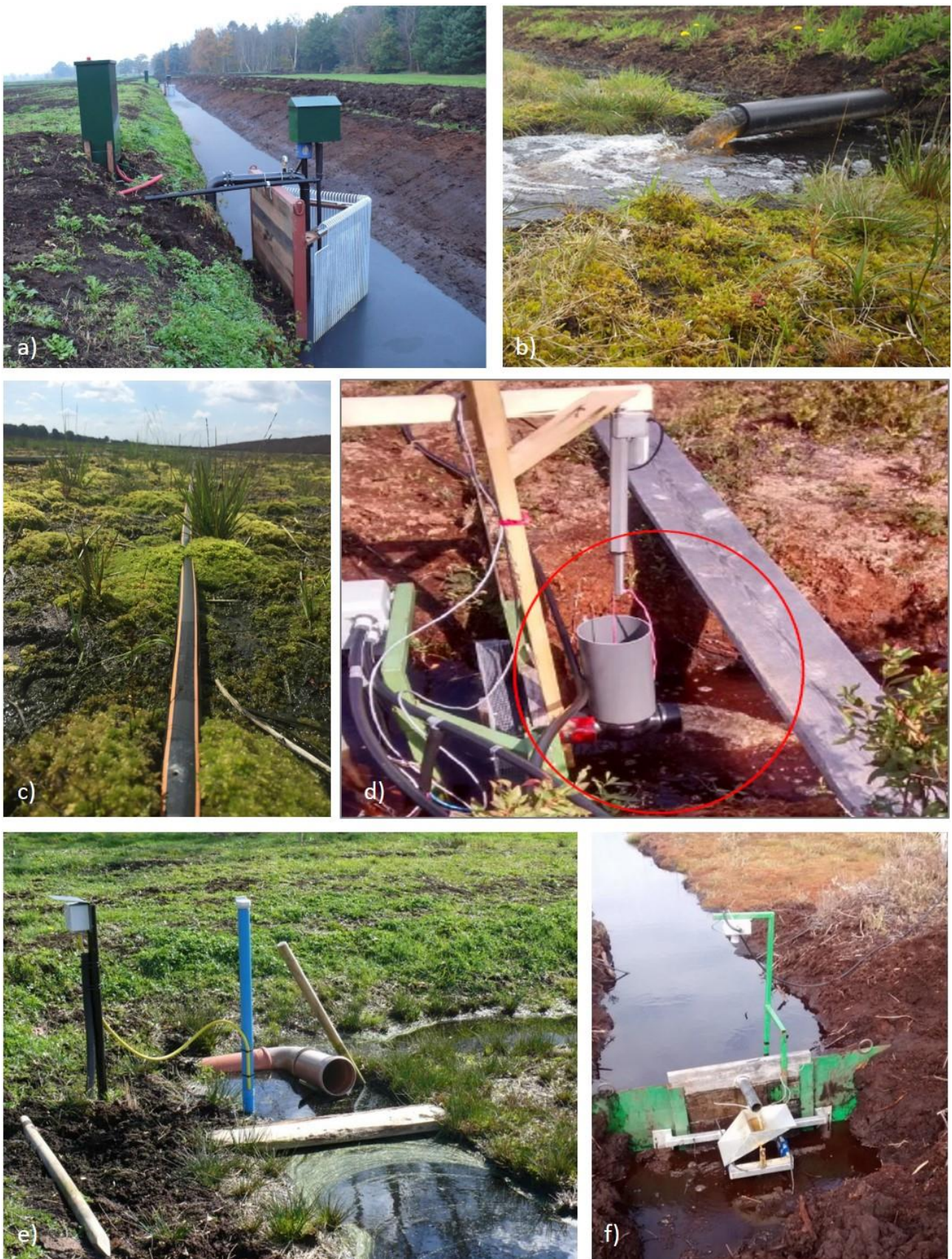
Figure 4. Water management components for Sphagnum farming sites: a) electric pump (Rastede); b) inlet into the irrigation ditches (Rastede); c) drip irrigation (Drenth); d) ‘adjustable ditch’ with an outlet (Shippagan 2); e) outlet with a data logger (Rastede); f) outlet (Saint-Modeste). Photos: a) and e) Sabine Wichmann, b) Greta Gaudig, c) Dorothea Rammes, d) and f) Peatland Ecology Research Group.
