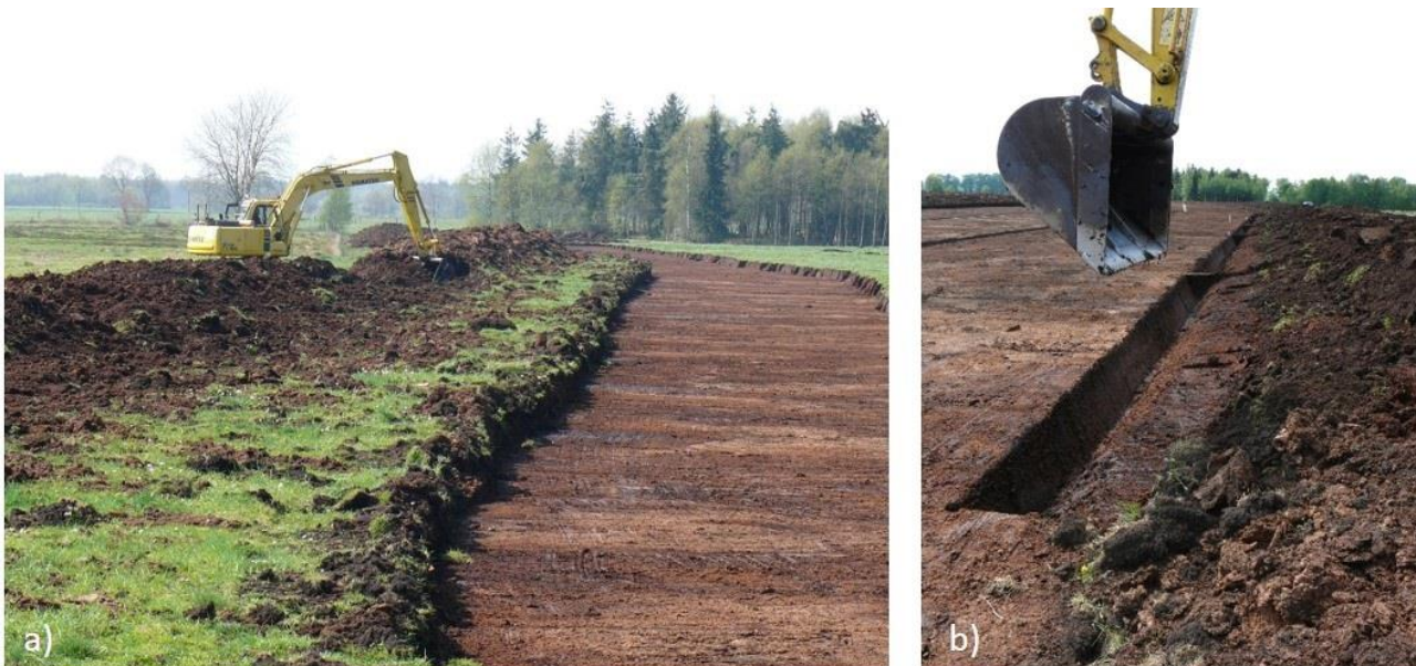
Figure 3. Setting up a Sphagnum farming site on former bog grassland in Germany (Rastede), using an excavator for a) removal of the degraded topsoil and b) construction of causeways and irrigation ditches. Photos: Sabine Wichmann.
