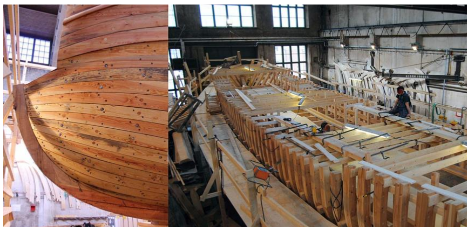
Figure 21. Shape of the hull and the construction process when using the skeleton-based technique: Finnish site.
