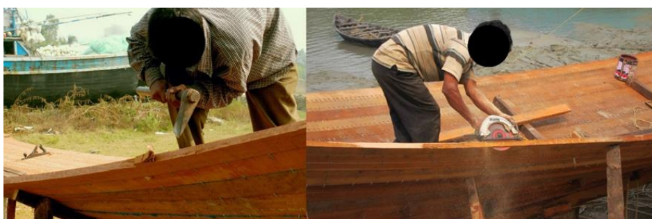
Figure 13. Installation of planks. Left: cutting the planks with an axe. Right: cutting the planks with an electric saw.
