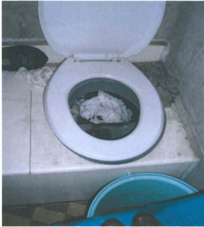
Plate 3.4: Urine diversion toilet showing faecal vault being used as a household waste bin
