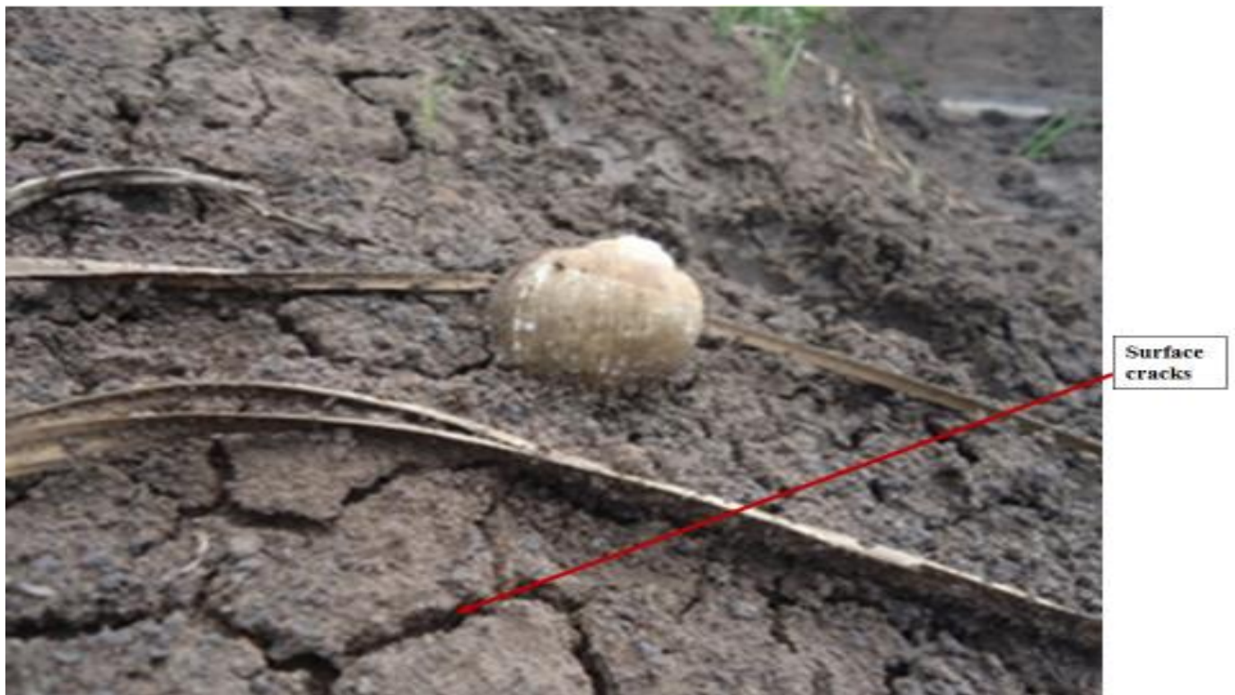
Fig. 4.12: Highly expansive materials with many surface cracks.
