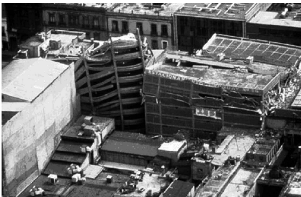
Photo 1. 1985's earthquake in Mexico: building collapse.
