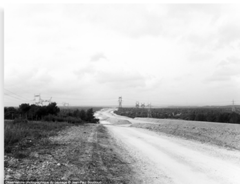
▲ Figure 25. Cabriès (Bouches-du-Rhône), chantier TGV, mars 1999. © J.-P. Bouilloud.
