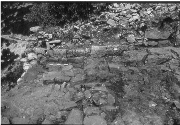
Figure 4: Rocca San Silvestro: The productive structures for the copper and the lead.
