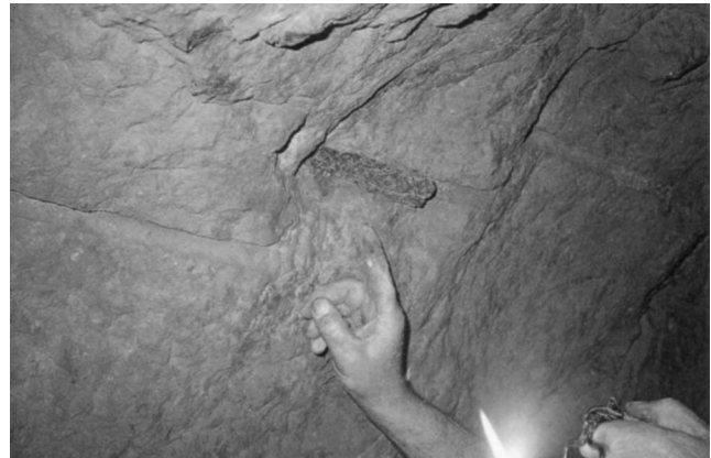
Figure 5: Earle shaft, 2nd level, traces of a manual starter on a gallery of mid-19th century.
