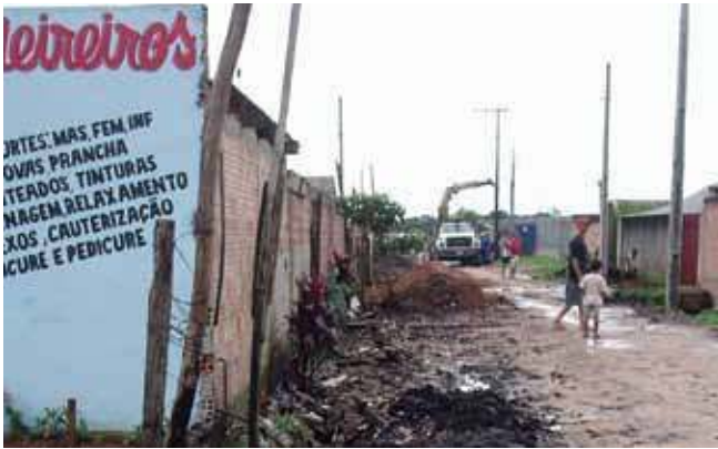
Makeshift Water Lines Improvised by Community Residents
