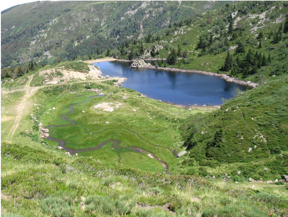
Figure 5 – Mountain reservoir partly built on a humid zone
